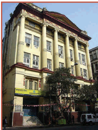
The building that housed the old James Finlay office in Kolkata
