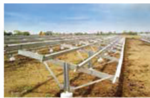
SOLAR MODULE MOUNTING STRUCTURE
