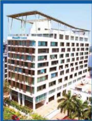
Stesalit Towers Our Corporate Headquarters at Kolkata
