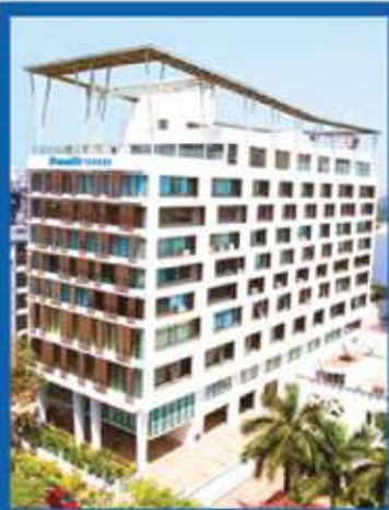
Stesalit Towers Our Corporate Headquarters at Kolkata
