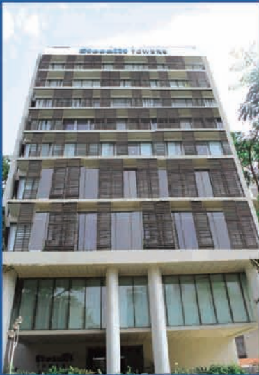
Stesalit Towers Our Corporate Headquarters at Kolkata
